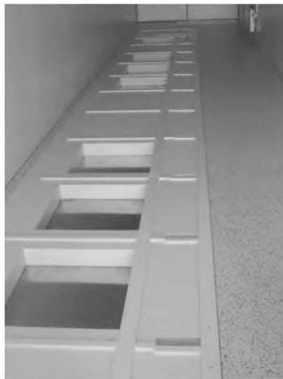
Sample picture of the floor inside enclosure.
